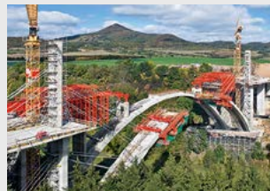
Bridge Formwork
